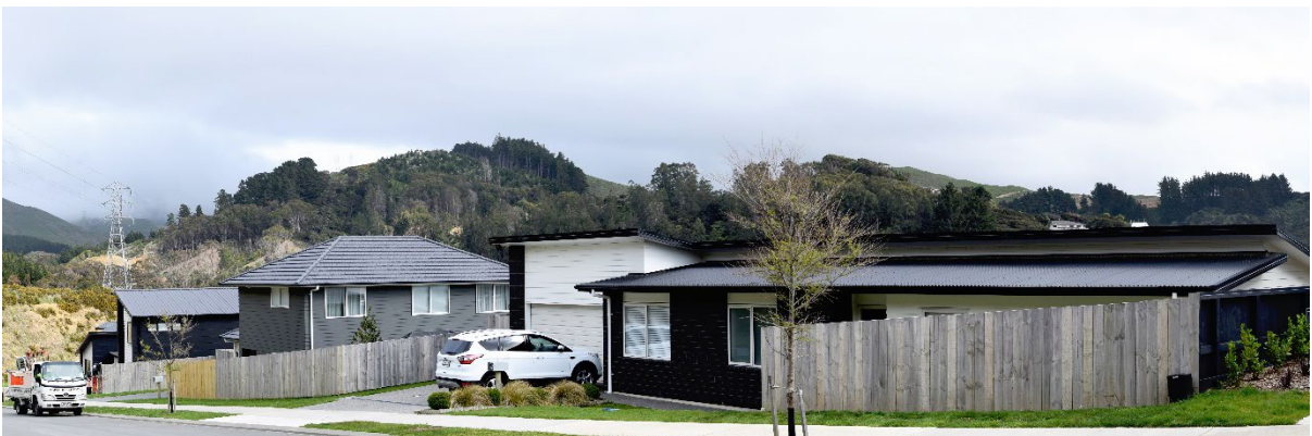
Figure 13: View 10 - of Lot 6 South, Lot 1 South, and Landcorp Lot from Navigation Drive, Whitby. The site is visible behind houses along Navigation Drive.
