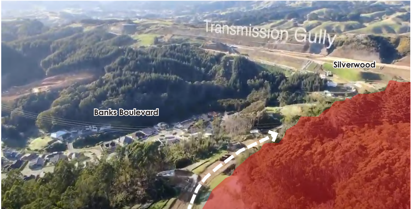
Looking north west across residential development on Banks Boulevard
