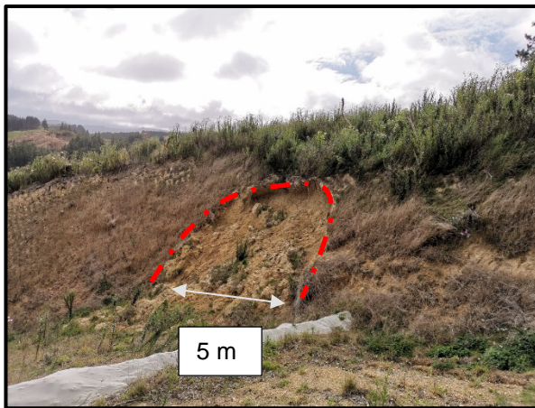
Photo 1: Slip scarp in access track cut.
