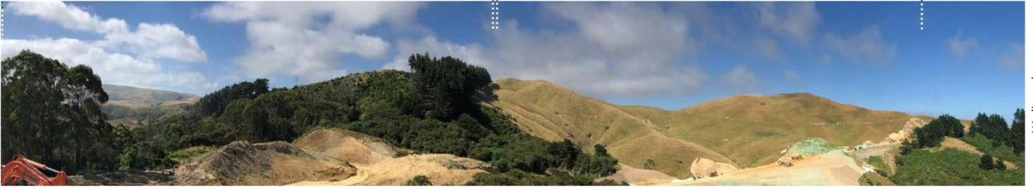
Looking from Waitangirua Link Road
