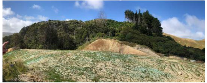
Looking south over Lot 6 from north side of Link
